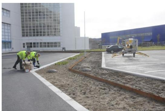
*Rainbed established as a demonstration and test of soil types, infiltration and vegetation.*
