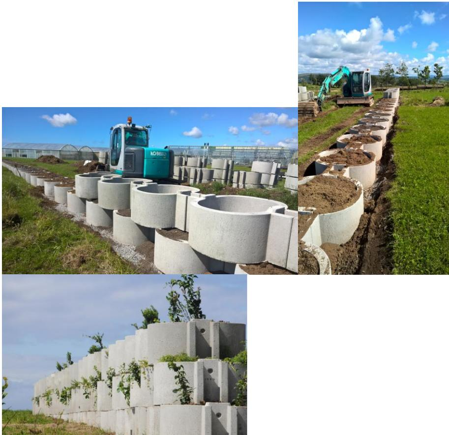
*Installation of a green wall (Skjæveland Wall) by Nibio Særheim. The plants are tested on both the sun exposed and shade side. The tests employ two soil types and the use of irrigation containers to support plant growth and resilience.*
